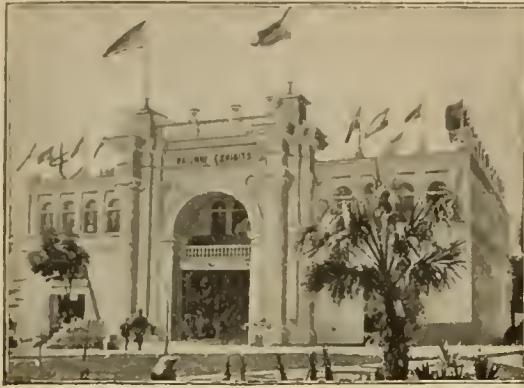
TERMINAL STATION, TENNESSEE CENTENNIAL.
